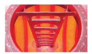
One example of a cost-saving innovation introduced by Greentank is the large-diameter tank bottom sump, which Greentank designed to eliminate the need and expense of a separate lift station when full use of a tanks capacity is necessary. The Greentank bottom sump provides that requirem ent while at the same time eliminating a potential source of leakage in the piping between a lift station and tank.
